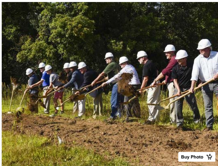
The first shovels of dirt were thrown during the groundbreaking for the new Tech High School Monday, Aug. 28, near 33rd Street South. (Photo: Jason Wachter, jwachter@stcloudtimes.com )
